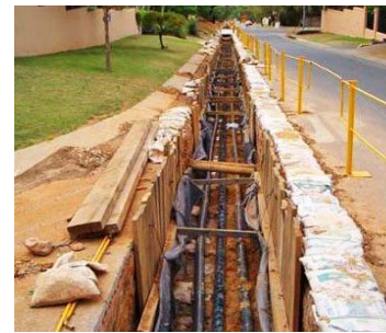
Integrated utility relocation
