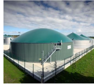
Biogas energy plant
